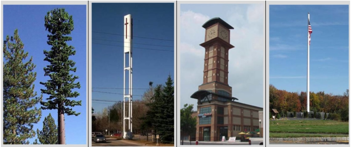
FIGURE 4.4.4.H.4.B: CONCEALED TELECOMMUNICATIONS TOWERS
