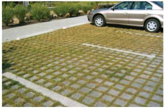
Incorporating stormwater management techniques into parking lots can include requiring landscaping and disallowing curbs and gutters so that water can flow into, not away from landscaped areas (left) and incentivizing the use of alternative pervious paving that allows water to permeate where it falls (right).
