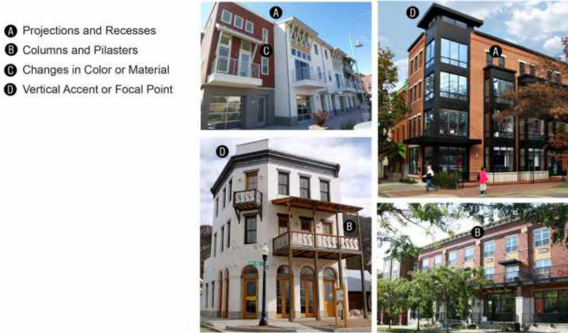
FIGURE 5.1.3.D.8: MIXED-USE BUILDING ARTICULATION
