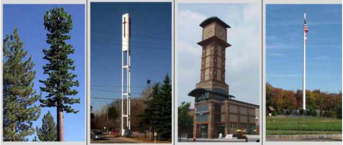
FIGURE 4.4.4.H.4.B: CONCEALED TELECOMMUNICATIONS TOWERS
