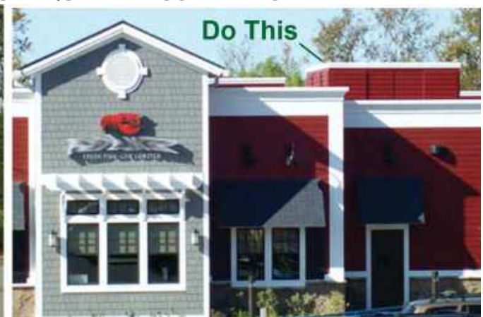
FIGURE 5.1.2.D.7: ROOFTOP EQUIPMENT SCREENING
